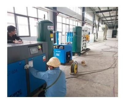
Innovative pressure swing adsorption (PSA) technology can be obtained through field gas system. PSA is a mature method of producing oxygen by using oxygen production system. Any company that buys two or one bottles of oxygen a week will benefit from the oxygen generator system (oxygen generator).
