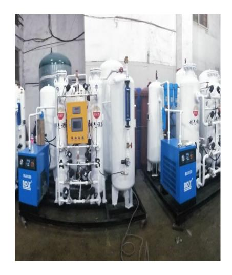
Suzhou XITE installed a 125 m3/h nitrogen generator for thermal cracking of tires with 99.5% purity and 5 KG/CM2 operating pressure.
