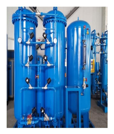
XITE Engineering Ltd. installed a 10 m3/h nitrogen generator for tire pyrolysis with 99.9% purity and 5 KG/CM2 operating pressure.
