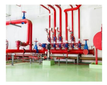
To mitigate the risk of fire outbreaks, building codes often require well-maintained fire sprinkler systems. Unfortunately, these fire protection systems are easily subject to corrosion from exposure to oxygen. To improve service life, the piping of sprinkler systems can be inerted using nitrogen. In this article, we will discuss how nitrogen generators can be used to enhance sprinkler systems.
