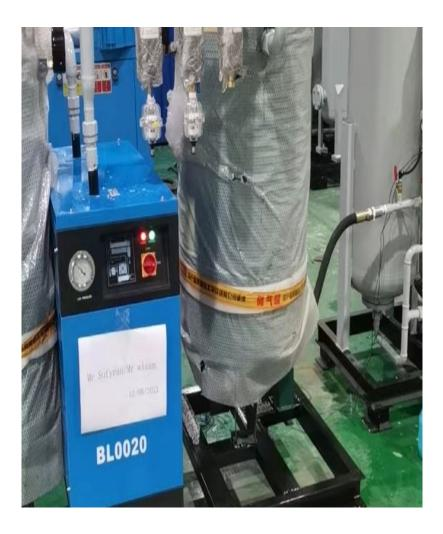
XITE Engineering Ltd. installed a 10 m3/h nitrogen generator for thermal cracking of tires with 99.5% purity and 5 KG/CM2 operating pressure.
