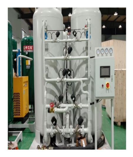
Suzhou XITE installed a 17 m3/h nitrogen generator with 98% purity and 6 KG/CM2 working pressure for the oil and gas industry.
