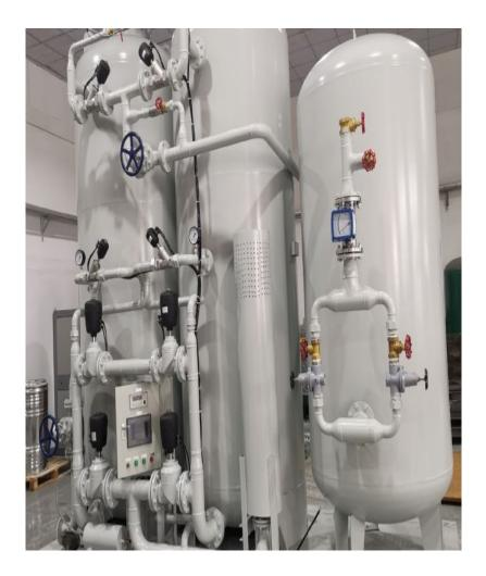
Suzhou Schitt has installed a nitrogen generator for annealing furnaces with a purity of 99.5%, a working pressure of 6 KG/CM2 and an annealing volume of 43 m3/h.
