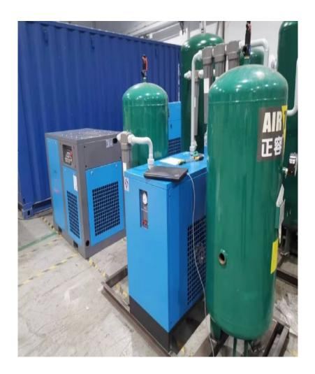
Suzhou XITE has installed a 50 m3/h nitrogen generator for food packaging with 99.9% purity and 6 KG/CM2 working pressure.
