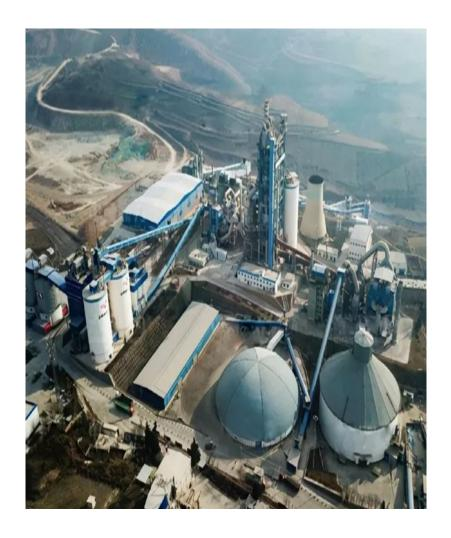
XITE supplied a nitrogen inert gas plant to a large cement manufacturing company in China. They needed nitrogen to clean coal mills, bag filters and coal bunkers to control fires due to spontaneous combustion of pulverized coal.
